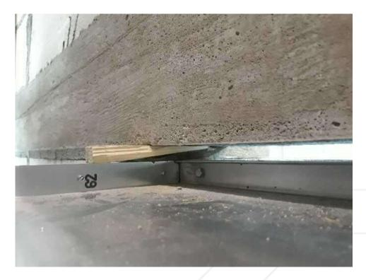
Figure 2. Correct preparation of the damper for installation (using mounting wedge)
